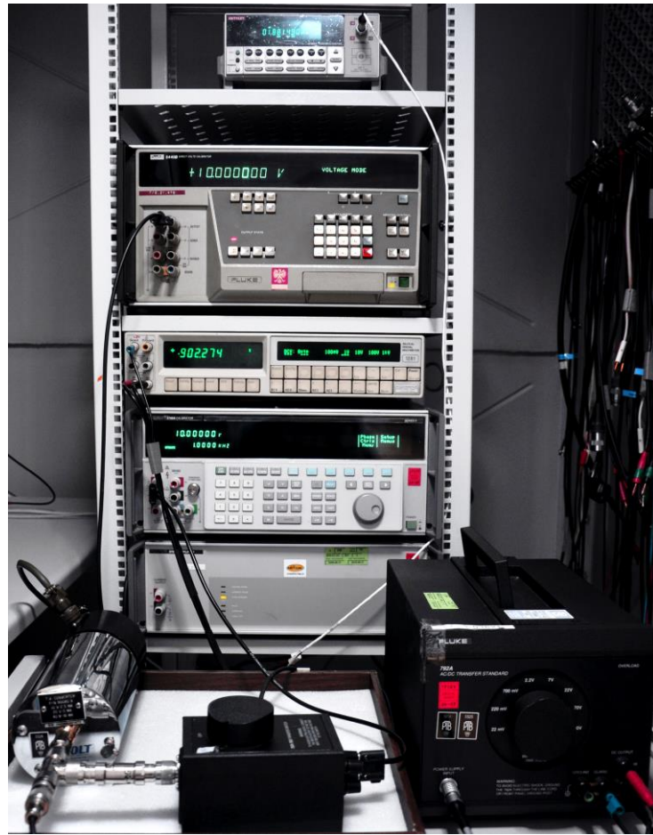
Fig. 9.6. AC-DC difference comparator system placed in GUM. The measuring station consists of: DC voltage source FLUKE 5440B calibrator, AC voltage sources FLUKE 5720A/5700A calibrator, Keithley 2182A nanovoltmeter, AC-DC Voltage Tee, reference converter HOLT model 11, UUT Fluke 792A.
